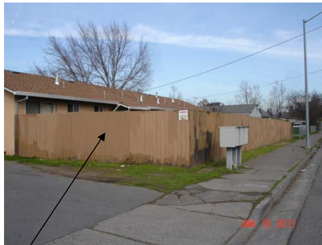
West facing portion (approx. 24'6")
