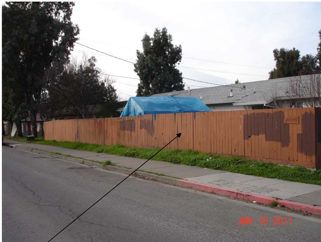
Main fence facing Aston Ave (approx. 86'4" long)
