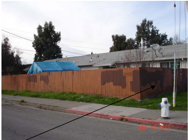
East facing portion (approx. 24'8")
